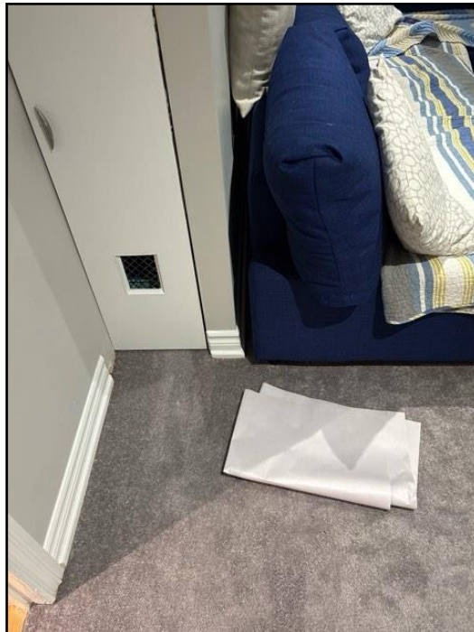
Floor drain not visible
