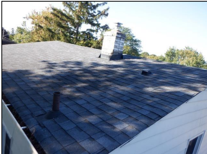
Asphalt shingles
