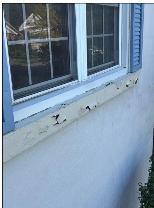
paint deteriorated
