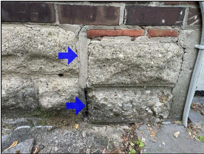
Mortar deterioration
