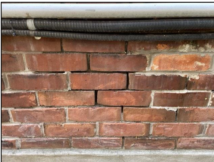
Mortar deterioration
