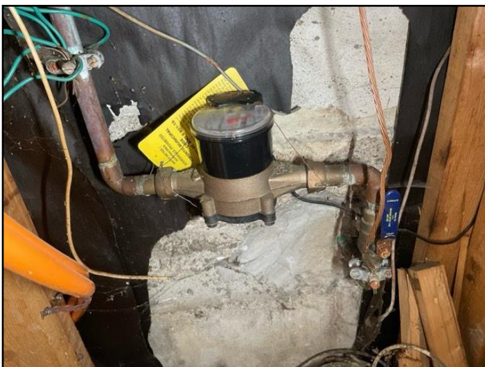
Front of the basement
