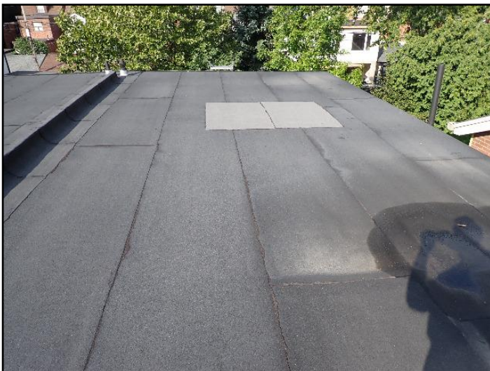
Upper flat roof
