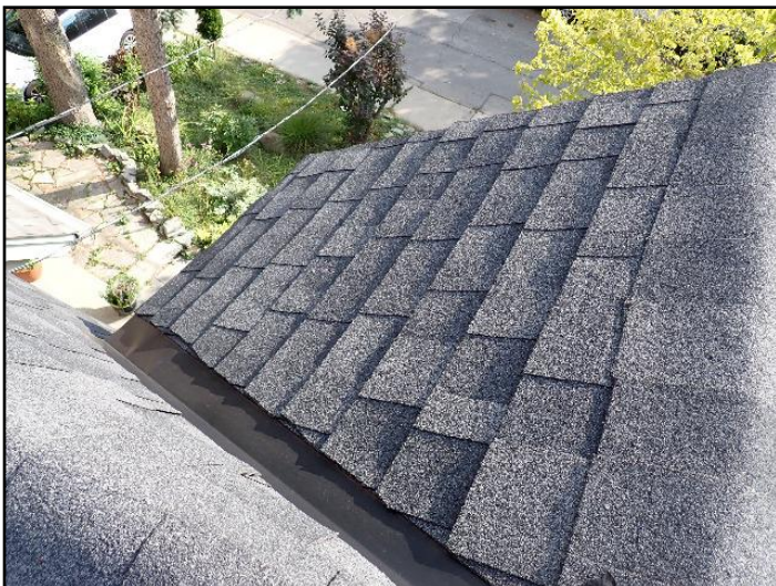
Asphalt shingles
